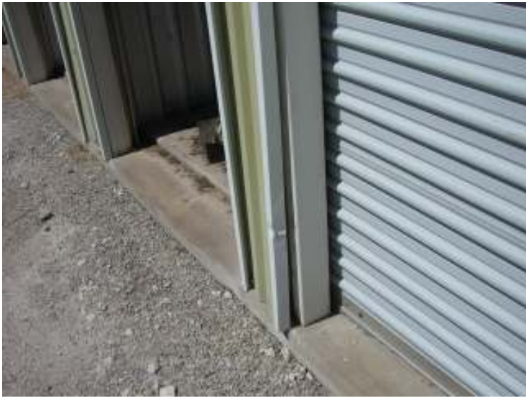
Unit 105 Has damaged door frame.
